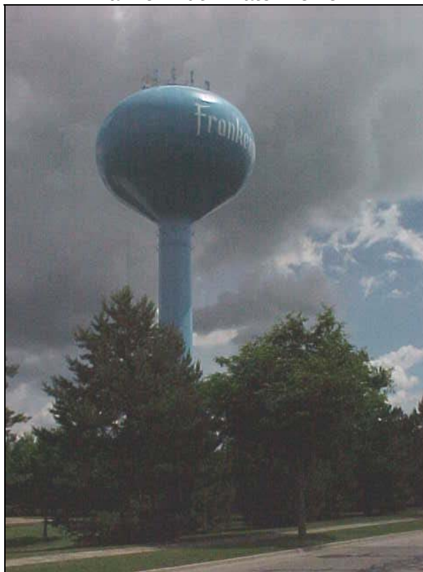
Photo 7-4 Frankenmuth Water Tower
