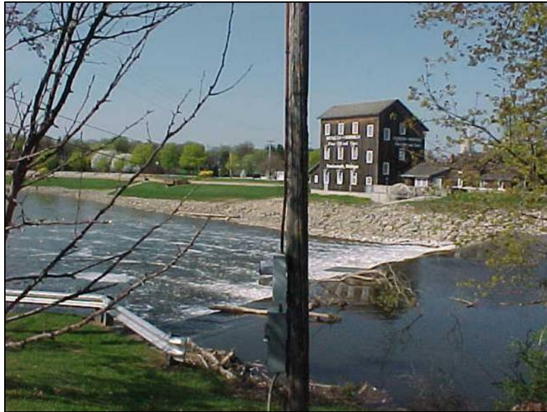
Photo 7-5 Cass River Dam
